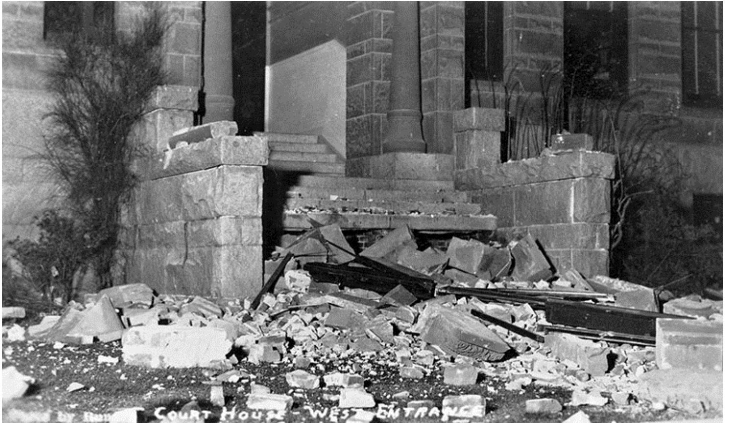
On March 10, 1933, a severe (approx. 6.4 on Richter scale) earthquake hit Orange County at 5:54 p.m. It was centered three and a half miles southwest of Newport Beach. Four Orange County residents were killed and many buildings were damaged or destroyed. (Including the Old County Courthouse above)
