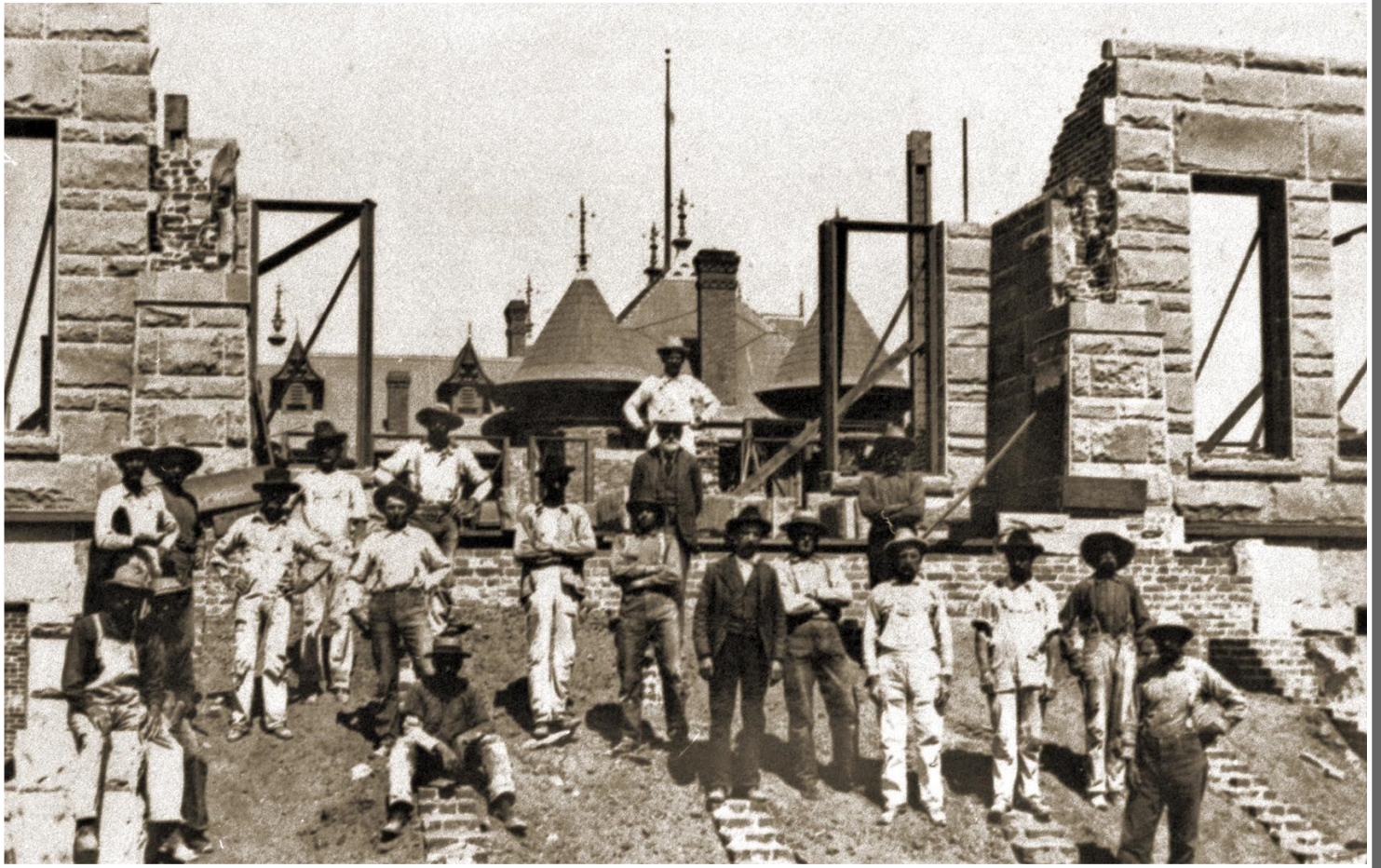
Construction workers pose on what would become the front steps of the (Old) Orange County Courthouse in 1900.
